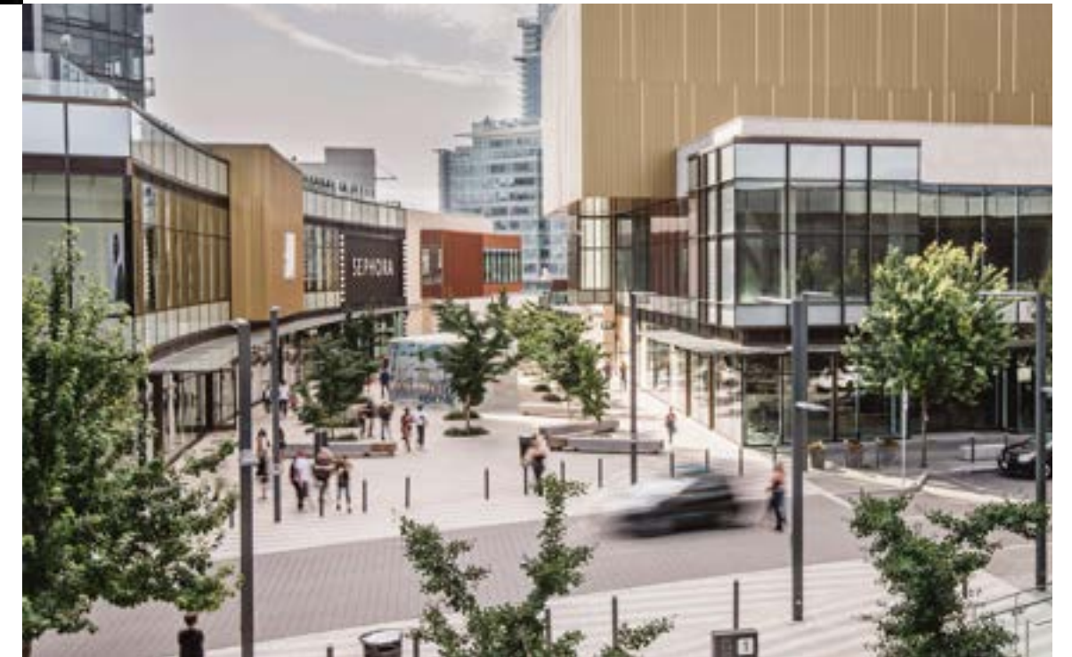
On-site maintenance and landscaping staff to keep the property flawless
